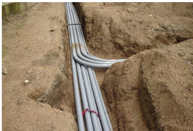
Fig. 5.24. Conduits installed underground
