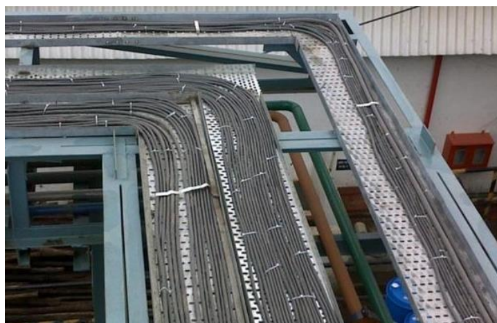
Fig. 5.28. Cable trays under the sealing of a facility
