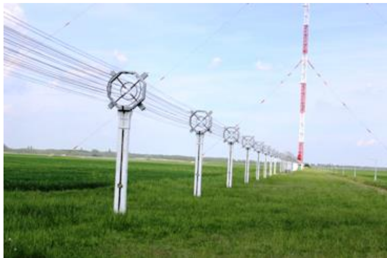
Fig. 5.5. Coaxial like arrangement feeding an antenna
