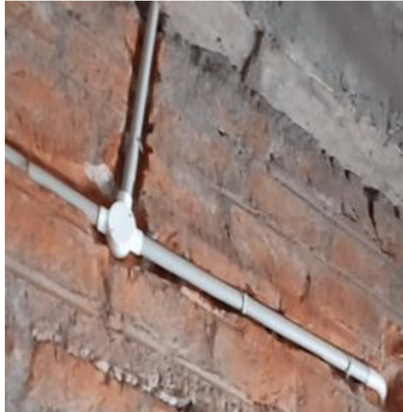
Fig. 5.22. Conduits installed into the wall
