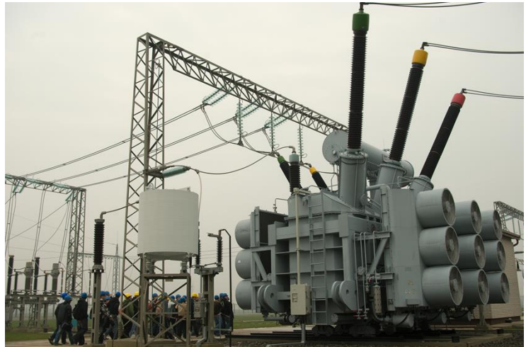
Fig. 3.2. Transformer (400/132 kV, 250 MVA)
