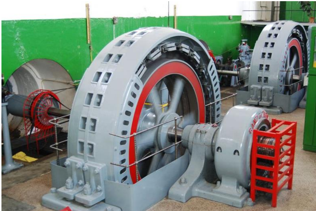
Fig. 2.14. The two hydro-generators in Gibárt having been operating since 1903
