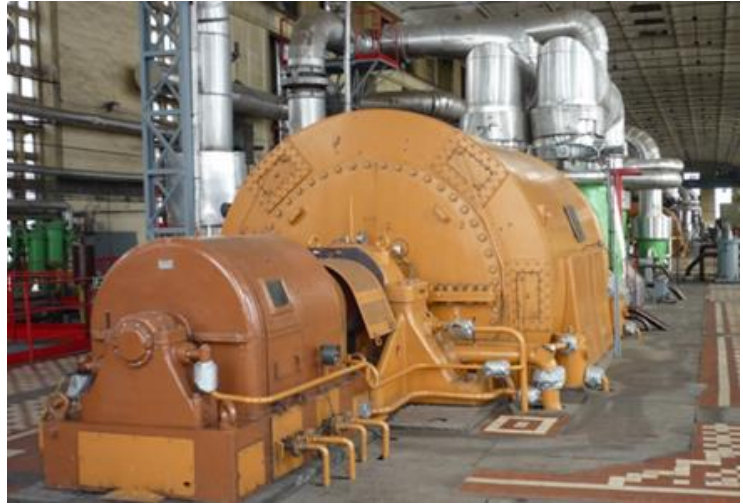
Fig. 3.1. Turbo-generator (source: PANNONPOWER)
