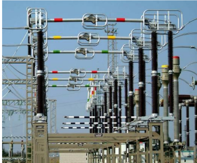
Fig. 3.6. 400 kV isolators
