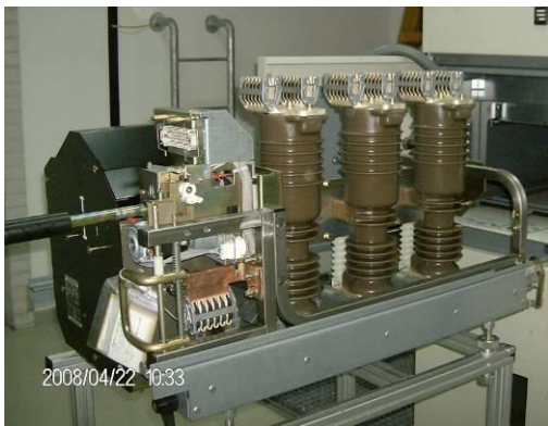
Fig. 3.11. Medium voltage circuit breaker (left), current transformer (middle) and a voltage transformer (right)
